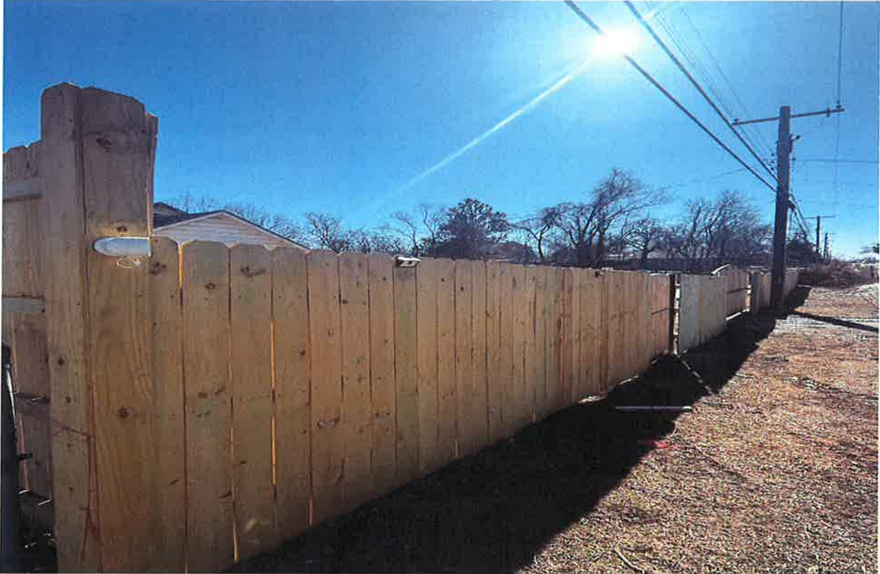
Fence placement relative to roadway and overhead utilities showing no obstruction
